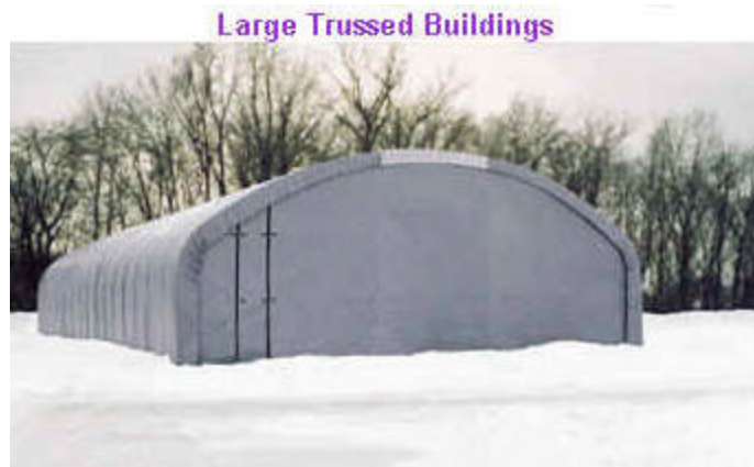
FIG1. View of the finished canvas building
